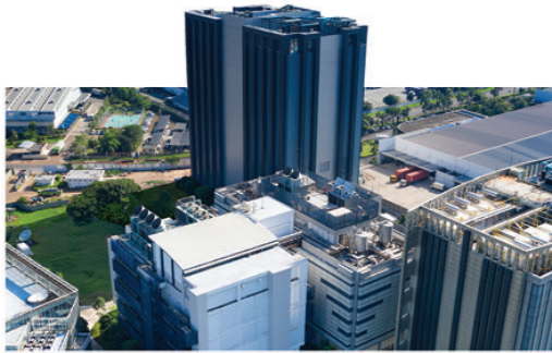
DCI-H1 CIBITUNG 4 DCs, 37 MW IT Capacity
