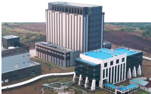
DCI-H2 KARAWANG 2 DCs, 27 MW IT Capacity
